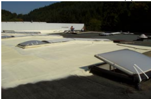
Figure 2 : Spray insulation on a flat roof and a round roof features and equipment
