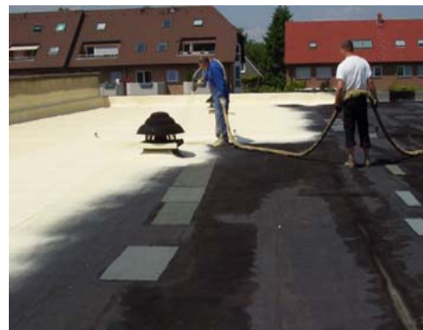
Figure 7 : Spray PU foam being applied on a flat roof
