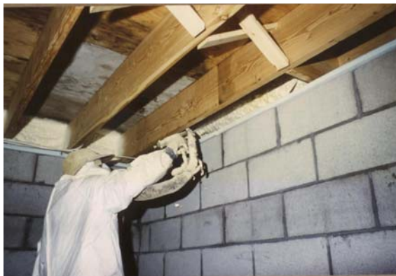
Figure 9: Spray foam being applied to insulate in between a wall and roof joists
