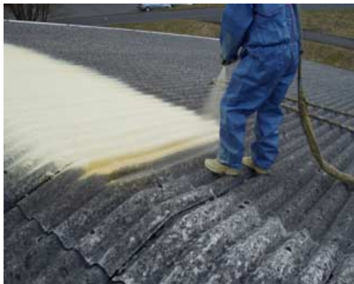
Figure 6 : Spray foam being applied to upgrade the insulation on a corrugated profile roof
