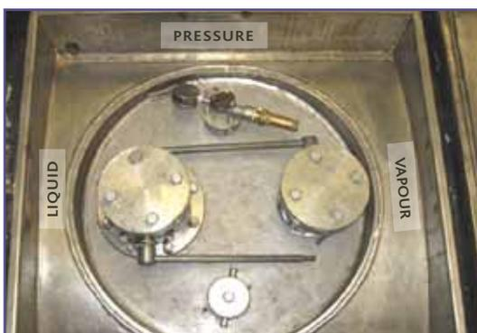
The dip pipe connection should be marked with "LIQUID" and the vapour return connection with "VAPOUR". Markings should be on an engraved plate as close as possible to the connection. It is recommended to also mark the air pressure connection (claw coupling) with "PRESSURE". As a minimum, the language on the engraved plates should be English.
